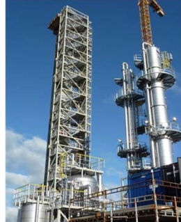
Technology Centre Mongstad, absorber and desorbers
